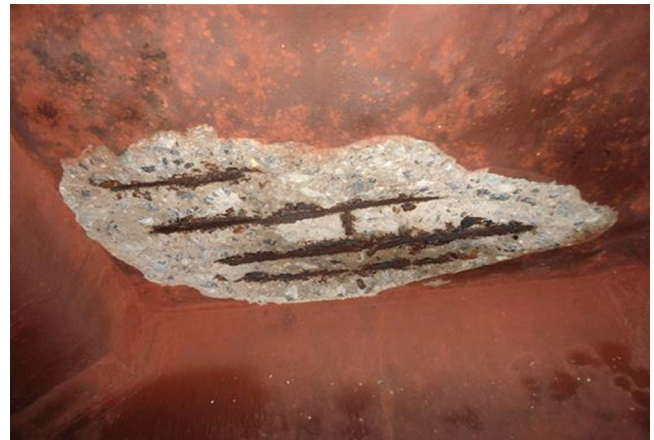
Figure 2. Panel corrosion condition.
