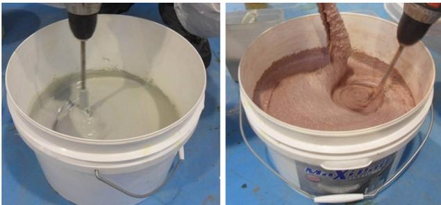
**Figure 2.** Mixing of grouts.
