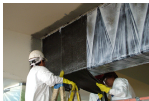
FIG. 2 APPLICATION OF EXTERNAL CFRP WRAP FOR REPAIRING A RC BEAM (with permission- http://www.fyfec.com ).
