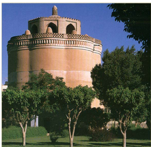
FIG. 3 KABOUTAR-KHANEH, A STRUCTURE MADE OF MALT-STRAW COMPOSITE IN THE 13th CENTURY, YAZD, IRAN.
