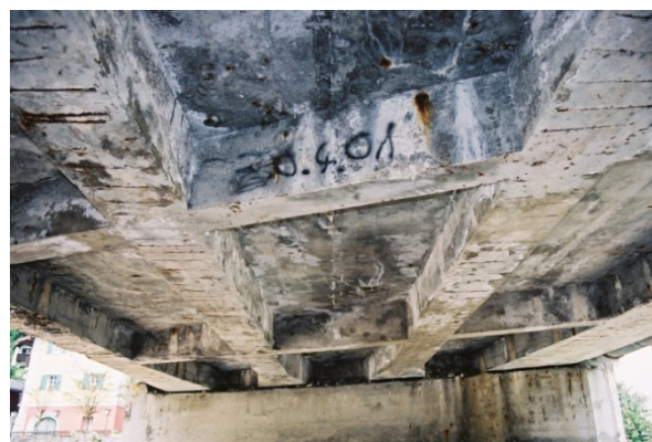
FIG. 1 EXAMPLE OF DAMAGED-DETERIORATED BRIDGE DECK (with permission- http://www.eng.cam.ac.uk ).
