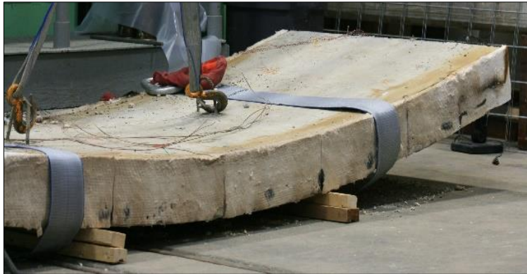
Figure 7. Excessive deflection of Slab-B.
